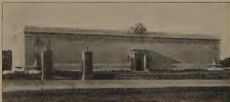
634 Willis Polk and Company, architects; photograph by Gabriel Moulin
